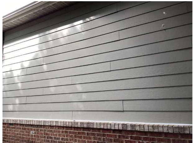
Fiber cement siding overview
