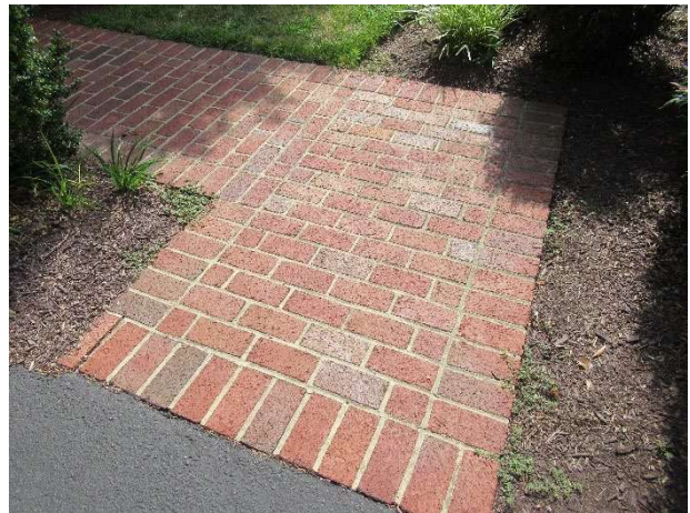
Masonry pavers overview
