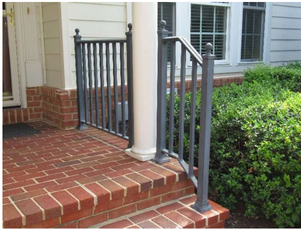
Metal railing overview
