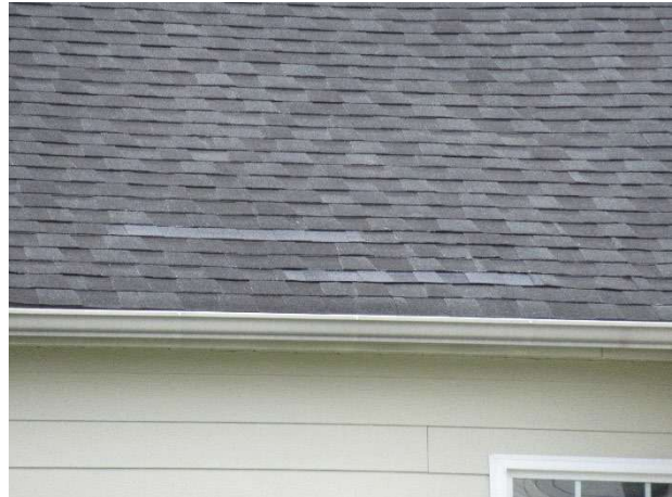
Partial replacements at townhome roof
