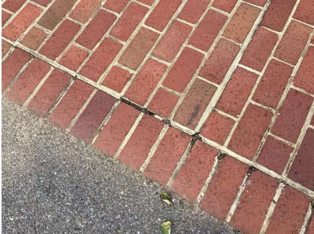
Mortar deterioration
