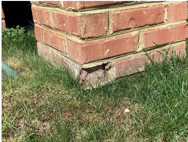
Masonry spall
