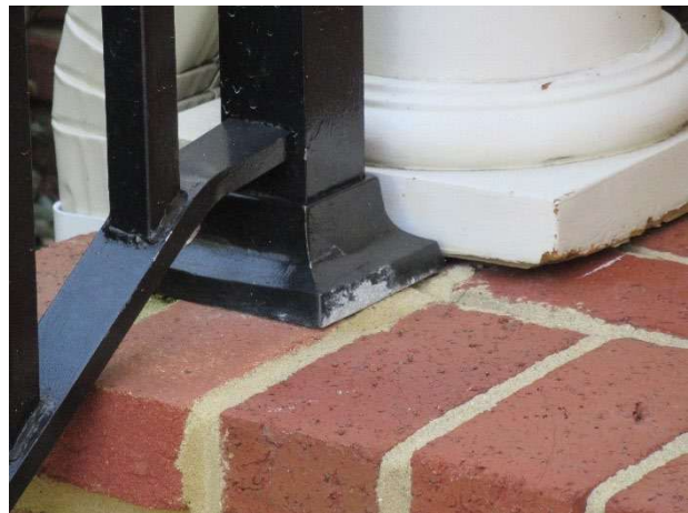
Finish deterioration
