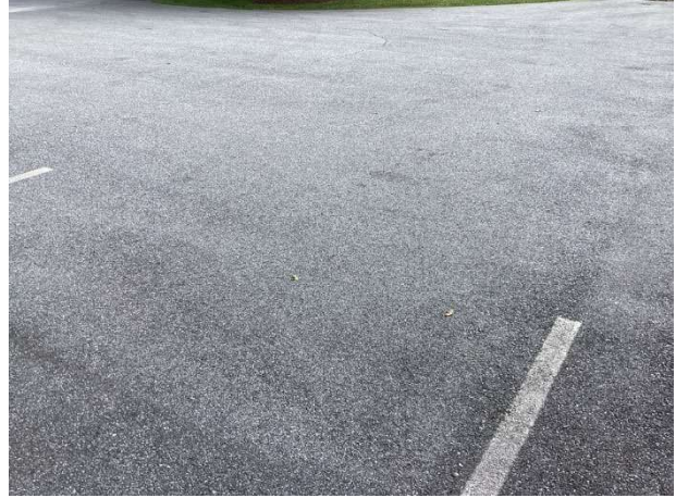
Asphalt pavement street and parking area overview
