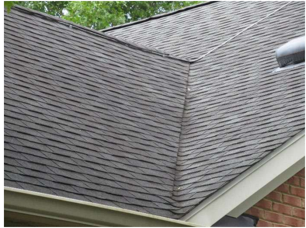
Asphalt shingle roof at clubhouse
