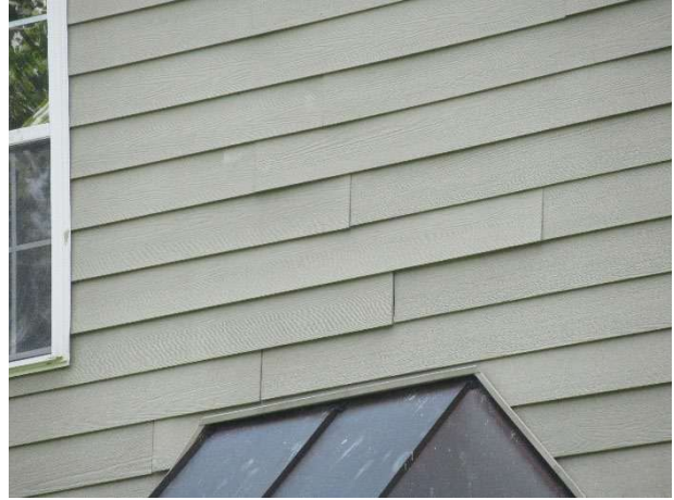
Warped siding
