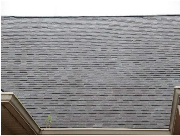
Asphalt shingle roof at clubhouse
