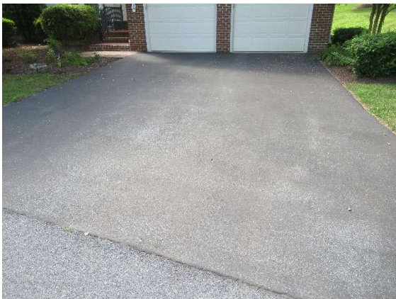
Asphalt pavement driveway overview
