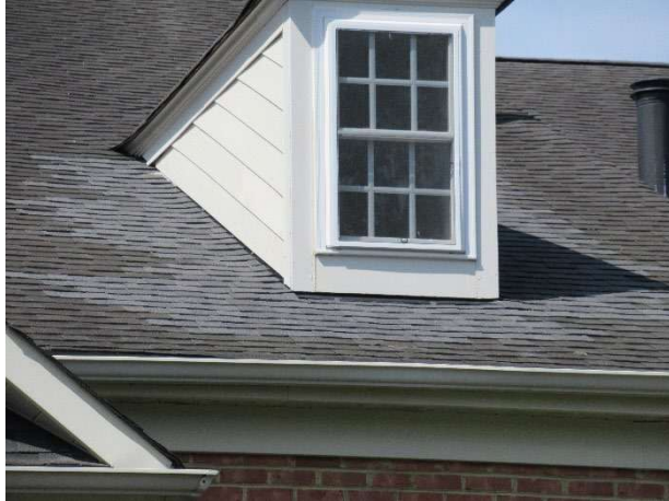
Partial replacements at townhome roof
