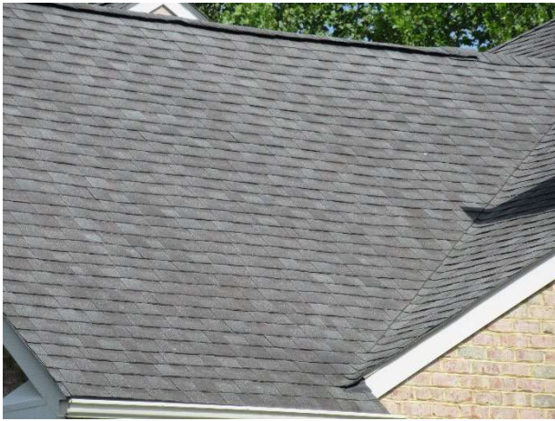
Asphalt shingle roof at single family home
