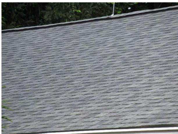
Asphalt shingle roof at wastewater treatment building
