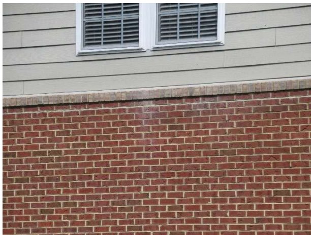
Efflorescence
