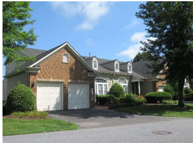
Townhome building front elevation overview
