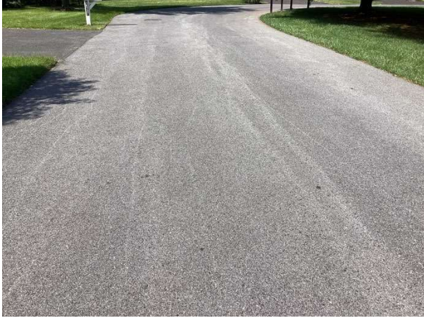
Asphalt pavement street overview
