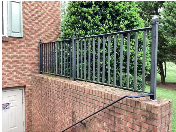
Metal railing overview
