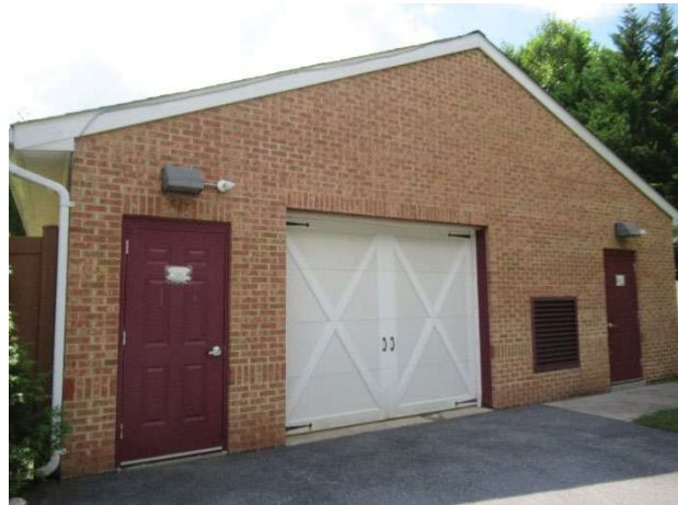
Wastewater treatment system building front elevation overview
