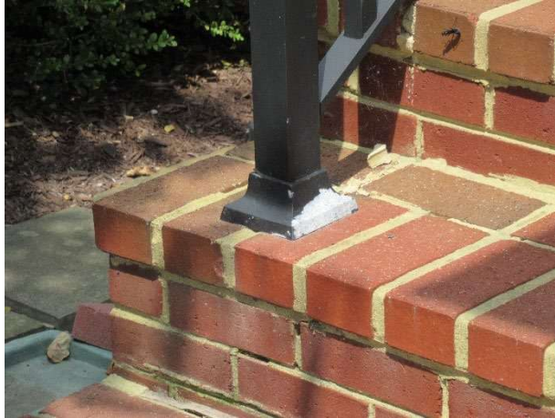
Finish deterioration
