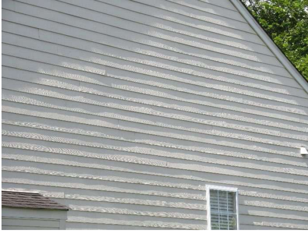
Warped siding
