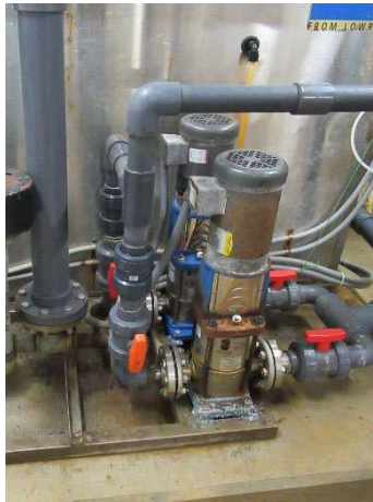
Repressurization pumps
