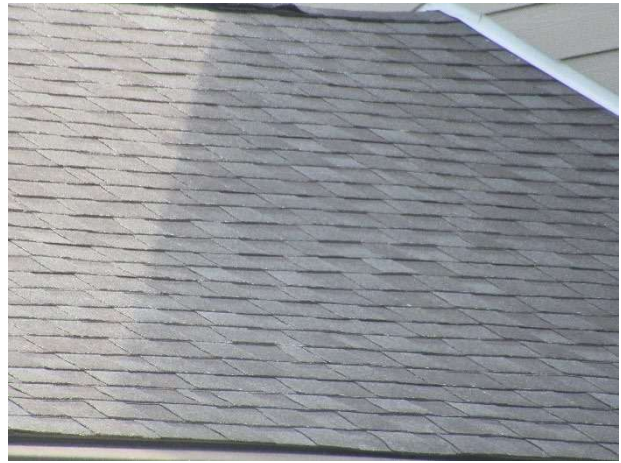
Asphalt shingle roof at single family home
