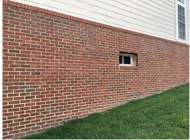
Masonry wall overview
