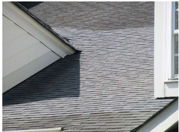
Partial replacements at townhome roof
