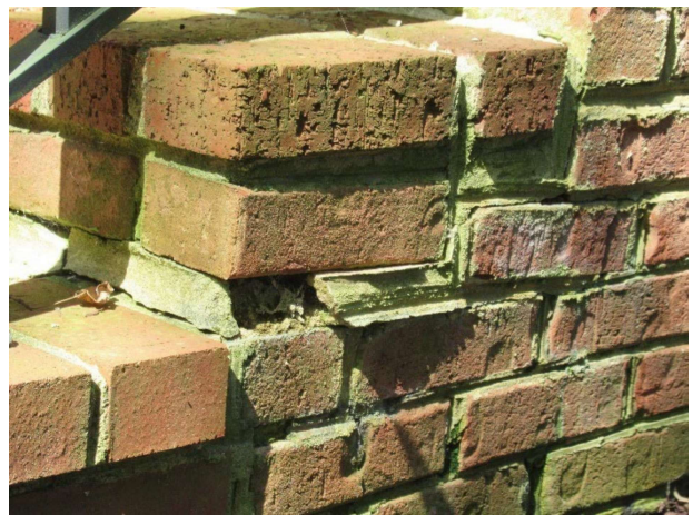
Mortar deterioration
