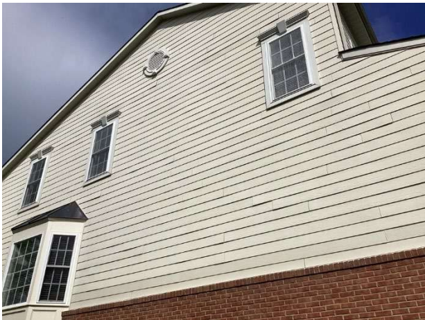
Fiber cement siding overview
