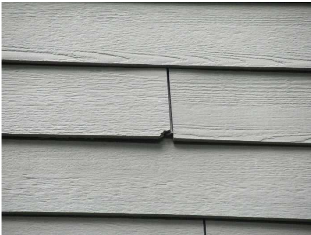
Siding damage
