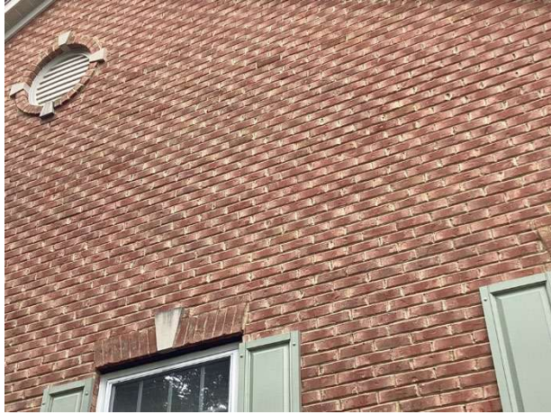
Masonry wall overview
