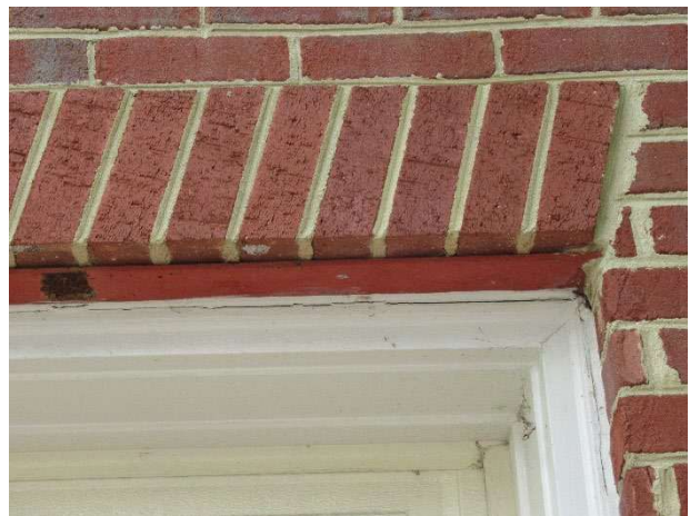
Sealant deterioration
