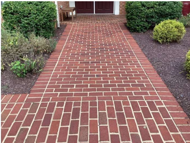
Masonry pavers overview
