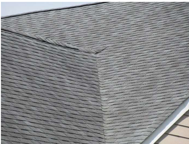
Asphalt shingle roof at single family home
