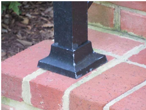
Finish deterioration
