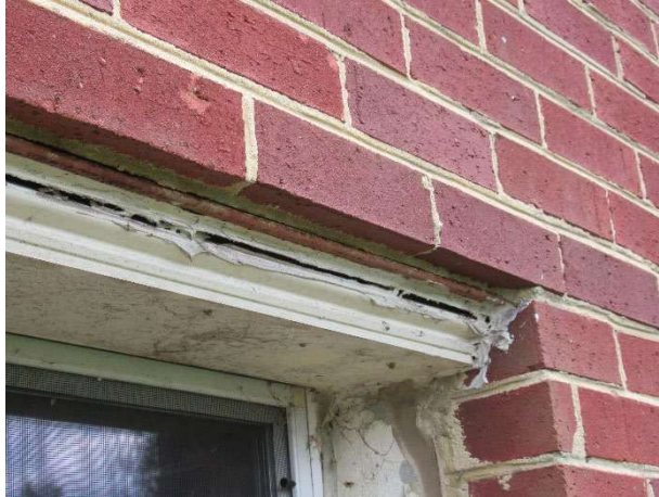
Sealant deterioration
